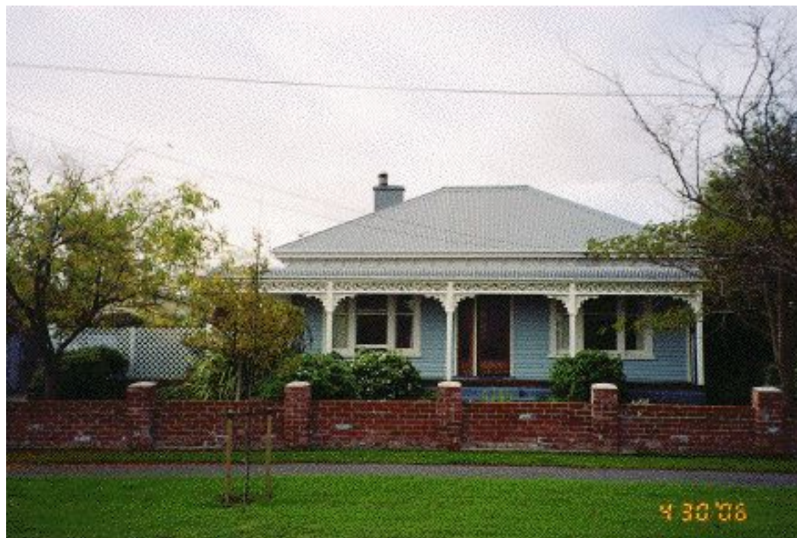
Photograph 2 - The home of Alfred and Harriett BADHAM at 11 Wildberry Street, Christchurch
